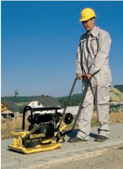
Compacting paving blocks with vulcolan mat
